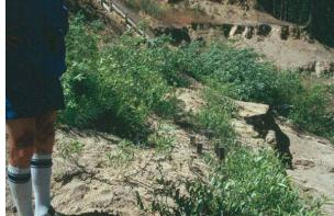
This brush box stabilized the toe of this slide even before the willow became established, and then vegetated the slide.
