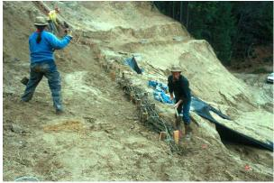
These brush boxes were installed for landslide repair. ("Old Faithful" cut slope project, Hwy 299W, CA, 1992)
