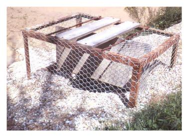
Figure 2. Drop inlet pipe with anti-vortex baffle and trash rack
