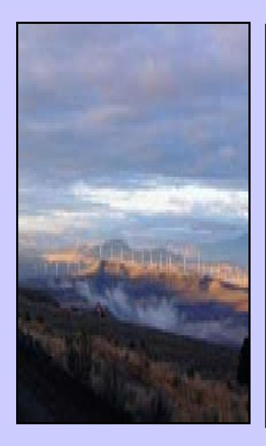
Elkhorn Valley Wind Farm spreads across the ridges of Pyles Canyon that run through Union County, Oregon. The site was chosen for its plentiful, steady winds and high-voltage transmission access. The wind farm consists of 61 Vestas V82 1.65 MW turbines and has an installed capacity of 101 MW - enough to power more than 30,000 Oregon homes with clean energy each year. Commercial operation began in the winter of 2007, and Idaho Power buys the wind farm's green energy.
